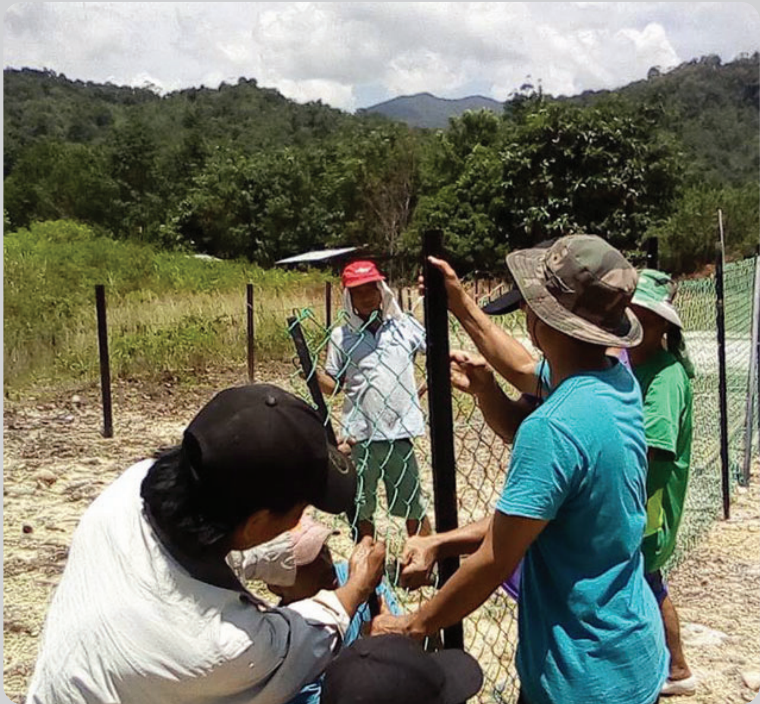
Above: Fencing at Buayan Hostel by villagers.
