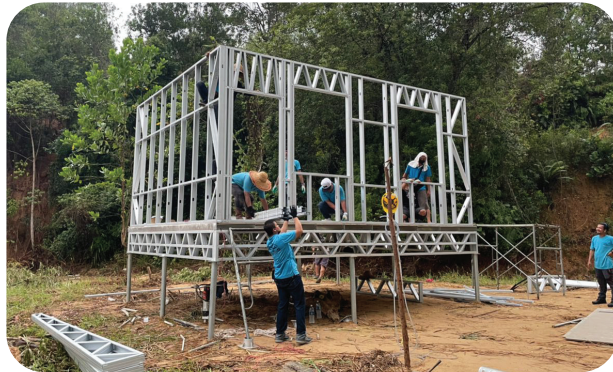
Before: In construction
